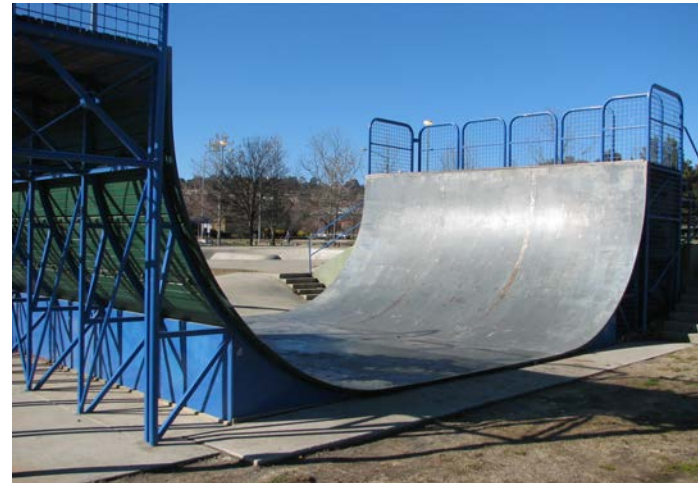
Image 2. Example of steel half pipes and large deep bowls typical of the 1980's
