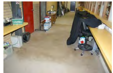
Image 6: extensive water damage from store room not water proof
