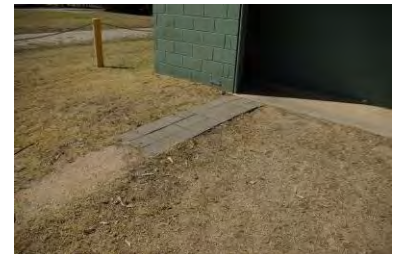
Image 3: Pathways to amenities are not to code / grade for BCA / DDA / AS 1428
