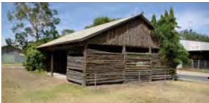
TIMBER 'LOG CABIN' PAVILION - IN POOR CONDITION - PRONE TO TERMITES - RECOMMEND TO BE DEMOLISHED.
