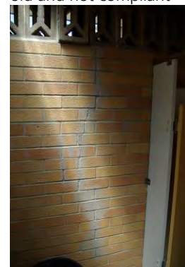
Image 12: major structural cracking evident
