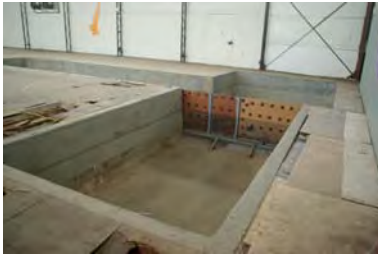
Image 4: Gymnastic pit – doesn't appear to be tanked (water proof)
