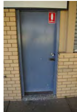
Image 3: Door hardware should be replaced with new
