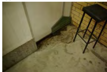
Image 8: Water damage evident around cool room. Further investigation is required.
