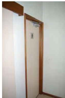
Image 2: All amenity signage not BCA / DDA compliant
