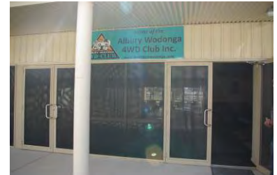
Image 3: Security mesh to all glazing and door ways
