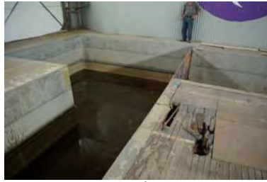
Image 5: Gym pits filled with water, not used, concrete/pits appear not be tanked
