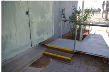
Image 7: Door / ramp landing not to AS 1428 requirements.
