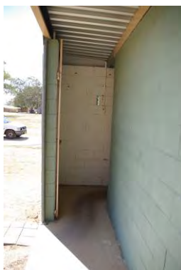
Image 4: Door width and landing are too narrow – under 1350mm – not compliant with BCA/DDA (AS1428.1)
