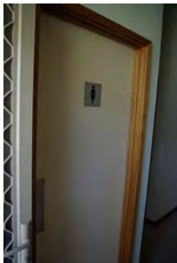
Image 1: All amenity signage not BCA / DDA compliant
