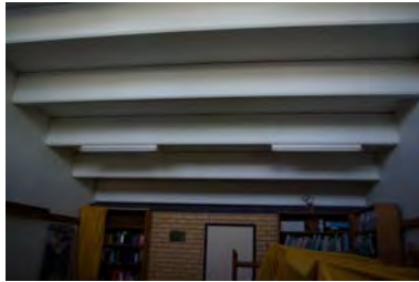
Image 7: no acoustic or thermal separation between room and underside of concrete grandstand
