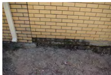
Image 11: Damp proof course may have failed or not installed at time of construction. Moisture or cold bridging associated with the cool room?
