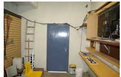
Image 9: No exit signage to path of egress. Not BCA compliant, including door hardware should be replaced with new
