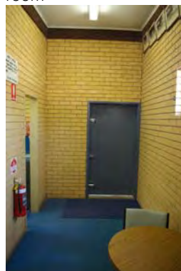
Image 5: No emergency egress signage and all door hardware not BCA compliant – can't escape from room
