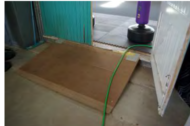
Image 8: internal access ramp into main hall space – too steep and not compliant to DDA/ AS 1428. In grade
