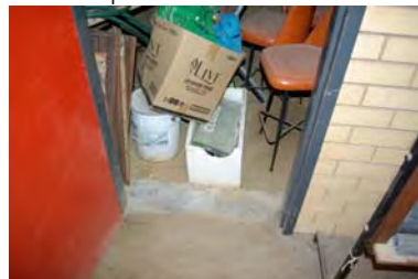
Image 8: floor of store is earth. Not evidence of water proofing or tanking of store room. Will always have water issues in building.
