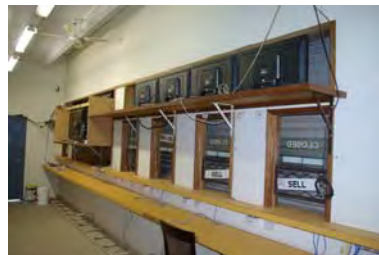
Image 5: exposed wiring not tagged or tied – potential WH+S issue
