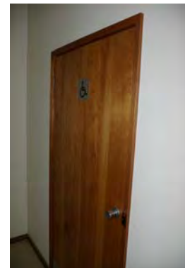
Image 3: Door access to accessible toilet – door width suitable however signage and door hardware not
