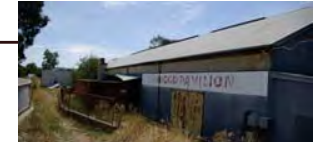
HEYWOOD PAVILION + POULTRY PAVILION - OVERALL BUILDING IN POOR CONDITION - RECOMMEND TO BE DEMOLISHED - EXTERNAL TOILETS NOT USED - INTERNAL FLOOR TO BE REMOVED - WATER INGRESS ISSUES TO SUB-BASE - ALL EXITS / EGRESS NOT 'BCA' COMPLIANT
