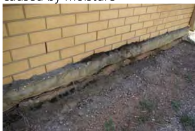
Image 10: Several areas show evidence of structural movement (cracking of masonry) and water damage
