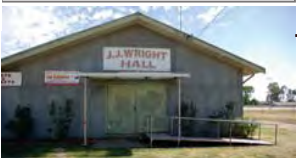
J.J. WRIGHT HALL - ACCESS TO PAVILIONS NOT 'DDA' COMPLIANT - ALL RAMP / DOOR ACCESS TO BE IMPROVED - BUILDING NOT SUITED FOR CURRENT TENANTS - OVERALL BUILDING IN FAIR CONDITION. NEEDS CONTINUAL MAINTENANCE WORKS.
