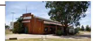
POINER HALL - OVERALL BUILDING IN REASONABLE CONDITION - RECOMMEND TO BE RETAINED + REFURBISHED - TOILETS TO BE UPGRADED AND COMPLIANT - EXISTING SIGNIFICANT TREE ADJACENT TO HALL TO BE RETAINED (UNLESS CREATING SIGNIFICANT DAMAGE TO BUILDING) - EXISTING PAVEMENT TO BE REINSTATE.
