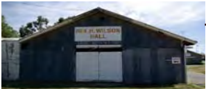
REX H. WILSON HALL - OVERALL BUILDING IN A FAIR CONDITION - SEVERAL WINDOWS REQUIRE UPGRADING - ACCESS / EGRESS NOT BCA COMPLIANT - NO EMERGENCY EXITS - GENERAL MAINTENANCE REQUIRED
