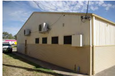
Image 2: Security mesh to all glazing and door ways
