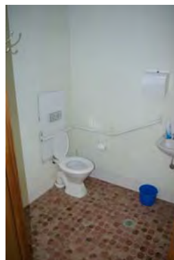
Image 5: Accessible room too small and basin too close to grab rail. Not BCA / DDA compliant
