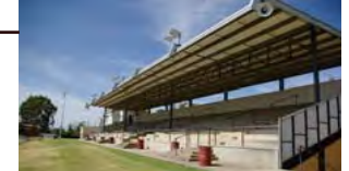
FRANK CORRIGAN GRANDSTAND - OVERALL IN GOOD CONDITION - MINOR STRUCTURAL ELEMENTS TO BE RECTIFIED - GENERAL MAINTENANCE REQUIRED. - CONSIDER SOLAR PANELS TO ROOF
