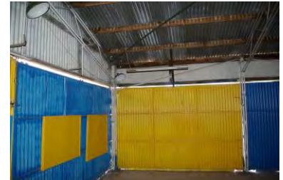
Image 3: No insulation to roof – basic roof construction
