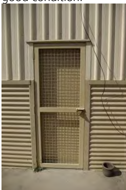
Image 7: Mesh door is not compliant for an egress door- pad locks not to be used.
