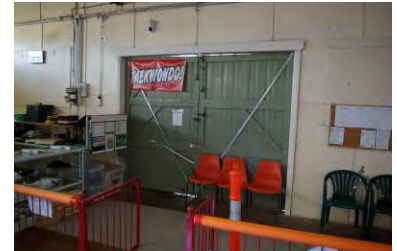
Image 9: Main entry door (double wooden) is not compliant for egress, door hardware and exit signage.
