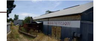
HEYWOOD PAVILION + POULTRY PAVILION - OVERALL BUILDING IN POOR CONDITION - RECOMMEND TO BE DEMOLISHED - EXTERNAL TOILETS NOT USED - INTERNAL FLOOR TO BE REMOVED - WATER INGRESS ISSUES TO SUB-BASE - ALL EXITS / EGRESS NOT 'BCA' COMPLIANT
