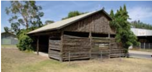
TIMBER 'LOG CABIN' PAVILION - IN POOR CONDITION - PRONE TO TERMITES - RECOMMEND TO BE DEMOLISHED.
