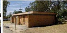
EXISTING TOILET BLOCK (BEHIND KIOSK) - OVERALL BUILDING IN POOR CONDITION - RECOMMEND TO BE DEMOLISHED - TOILETS NOT FIT FOR PURPOSE - NO 'DDA' / BCA ACCESSIBLE AMENITIES - ALL EXITS / EGRESS NOT 'BCA' COMPLIANT
