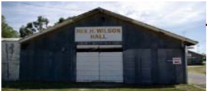
REX H. WILSON HALL - OVERALL BUILDING IN A FAIR CONDITION - SEVERAL WINDOWS REQUIRE UPGRADING - ACCESS / EGRESS NOT BCA COMPLIANT - NO EMERGENCY EXITS - GENERAL MAINTENANCE REQUIRED
