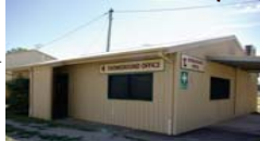
KD WATSON HALL + SHOWGROUND OFFICE - OVERALL BOTH BUILDINGS IN GOOD CONDITION - INSIDE TOILETS NEED TO BE UPGRADE TO MEET BCA + 'DDA' COMPLIANCE - EXIT / EGRESS DOORS TO BE BCA COMPLIANT, AS DOORS CAN'T BE LOCKED WITH STEEL MESH GATES.
