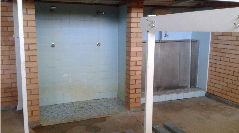
The showers and toilet facilities require upgrades, hot water added, the floors to be resurfaced and lights installed to the cubicles.
