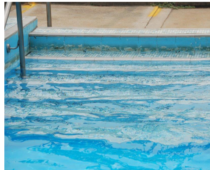
There are steps and a handrail into the big pool, however, the rail is too high.
