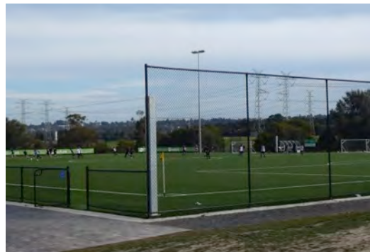
Image 3. Example (3) of permanent perimeter sports field fencing
