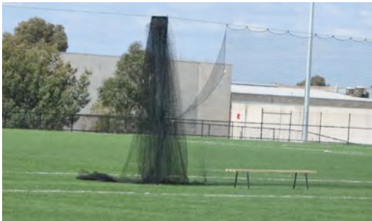
Image 5. Example (5) field divider netting supported by overhead cable as in previous photo, with netting drawn open
