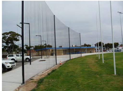
Image 2. Example (2) of permanent perimeter sports field netting
