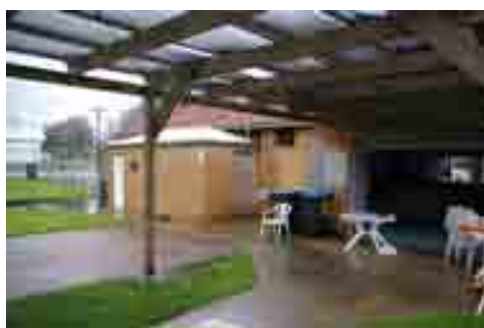
14) First aid room – not clearly accessible from pools – poor location for signage.
