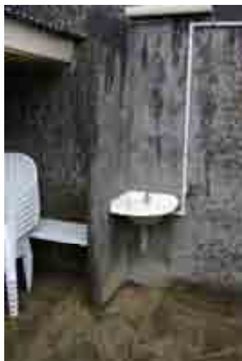
17) Typical steel basin with exposed plumbing.
