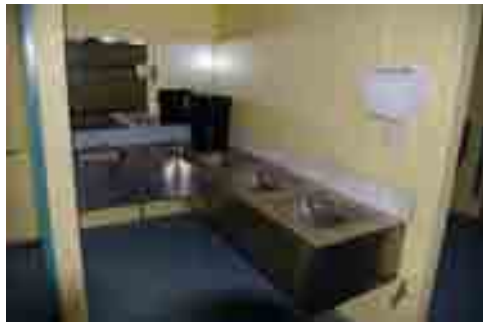
24) Stainless steel wall mounted basins to female change – too close and restricted. 25) Typical pan in change rooms.
