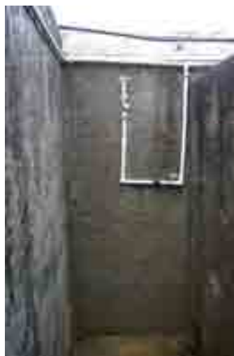
18) Typical condition of showers. Shower rose may be water saving but pipe work – very poor.
